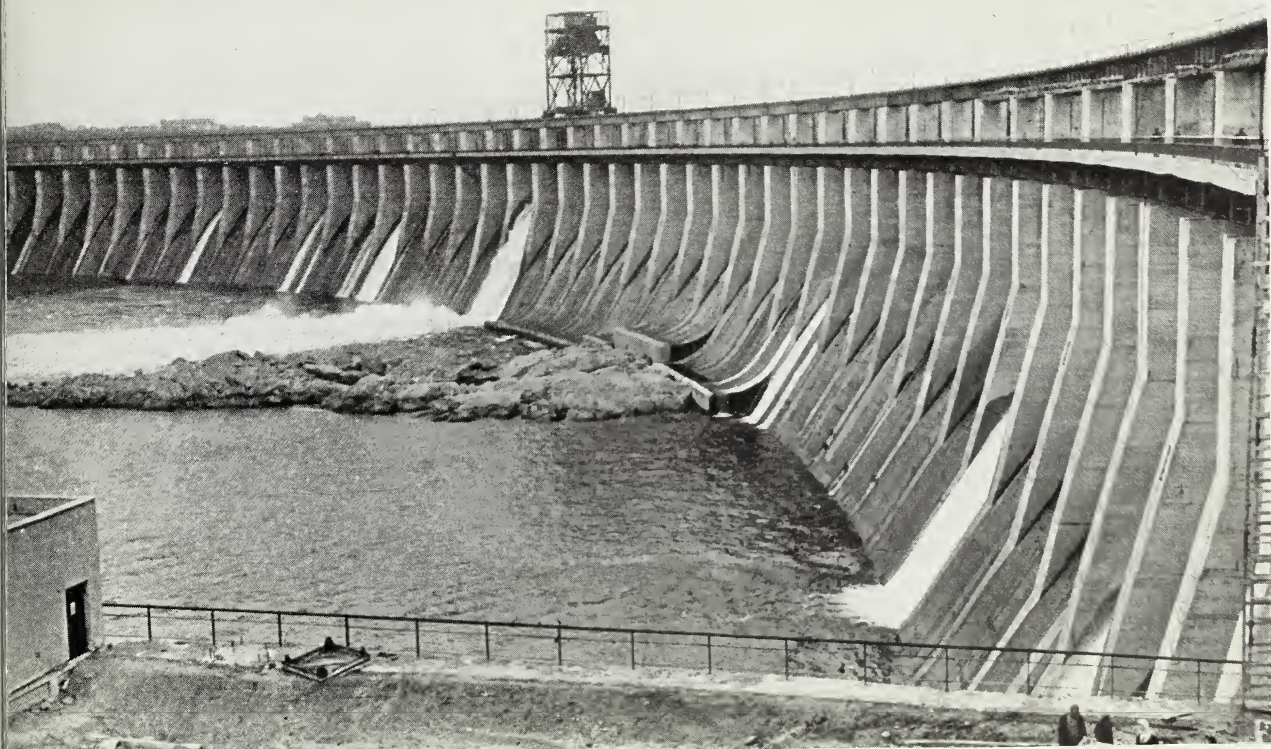
THE GREAT DAM AT DNEPROPETROVSK
